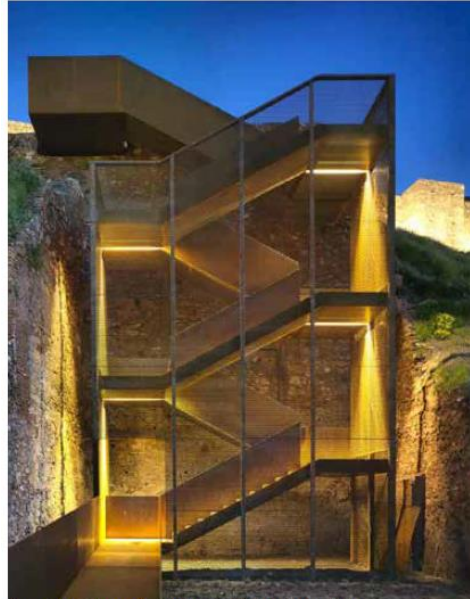
Figure 2.08: New corten walkway and steps inserted into Roman ruins, Malaga (OAM Arquitectos)
